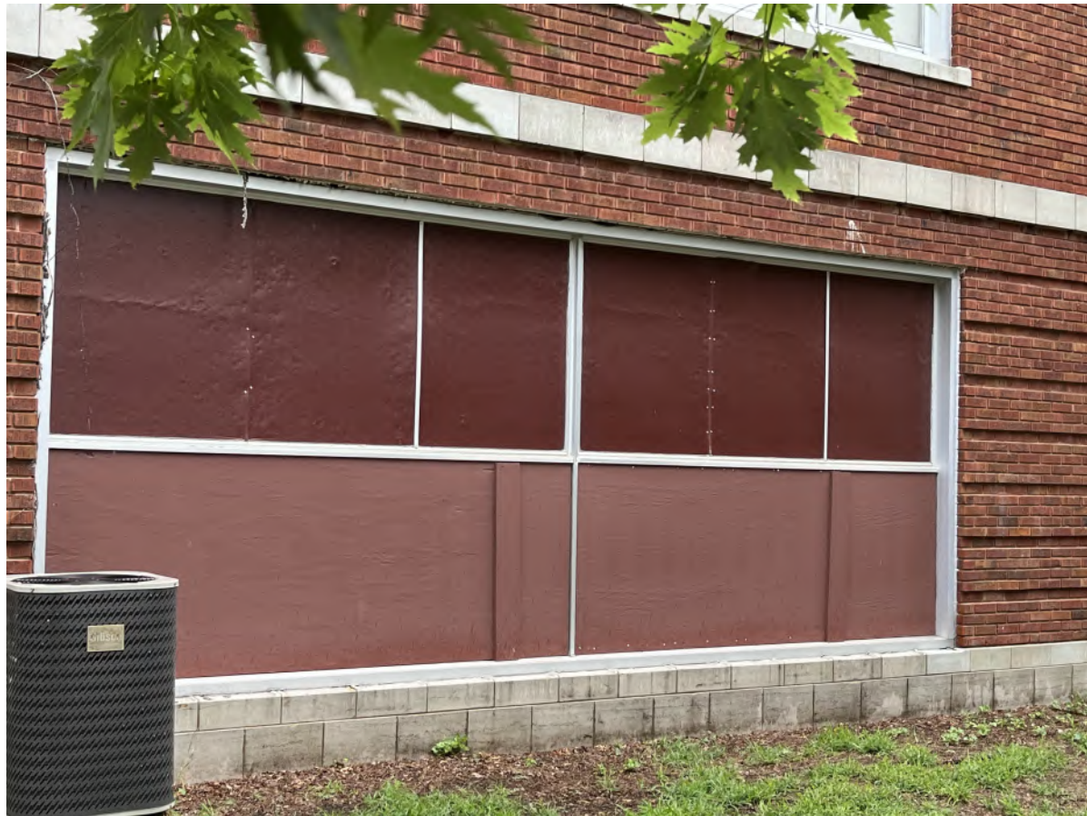
Photo 9. Representative window assembly for Unit Price Item No. 9. Approximate dimensions: 20 feet × 9 feet. Unit price shall be applied on a per-window basis only when authorized by the Owner and/or Atlas. Removal includes the metal window frame, asbestos-containing glazing compound, and asbestos-containing perimeter caulking.
