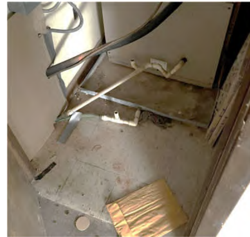
Photo 8: Floor tile in a 2 nd floor HVAC closet, included in the asbestos abatement scope.
