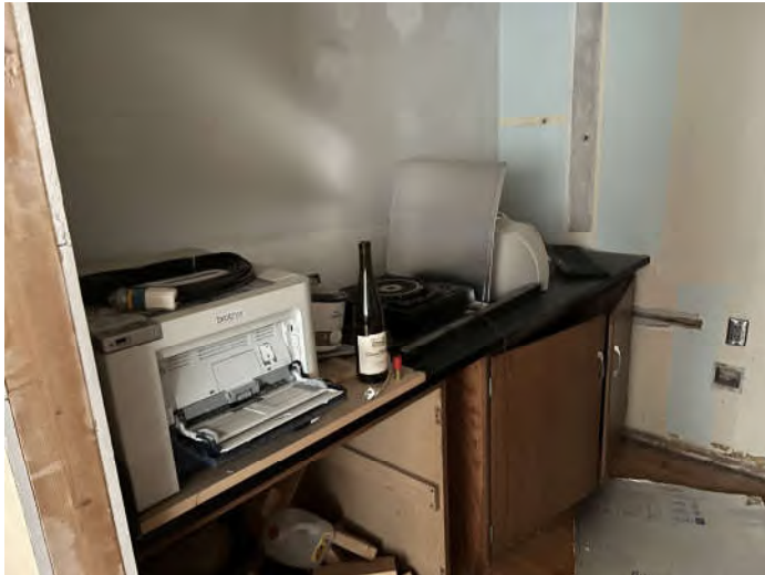
Photo 5: Countertop identified for removal as part of the asbestos abatement scope.
