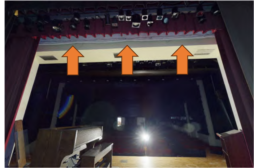
Photo 2: White rolled up fire curtain above the stage, included in the asbestos abatement scope.
