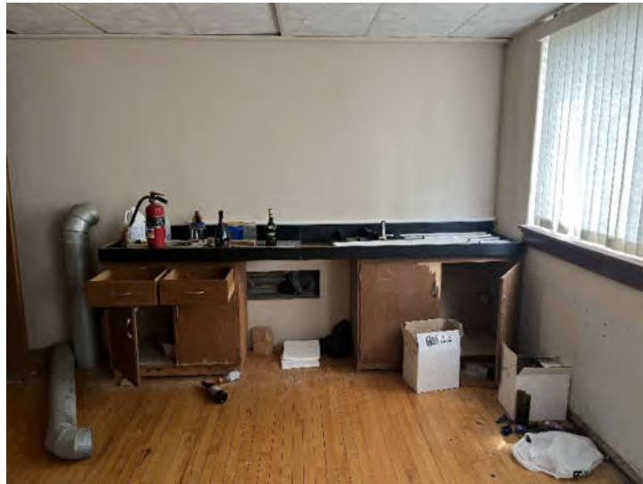
Photo 3: Countertop identified for removal as part of the asbestos abatement scope.
