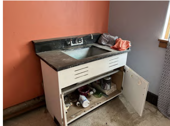
Photo 6: Countertop identified for removal as part of the asbestos abatement scope.
