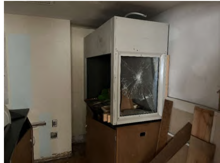
Photo 4: Fume hood identified for removal as part of the asbestos abatement scope.
